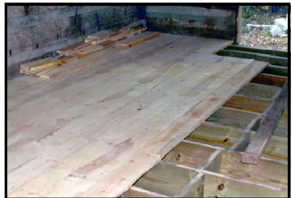
Installation of the "floating floor"
